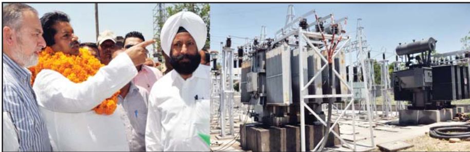
Minister for Housing Raman Bhalla inspecting newly upgraded receiving station at Sainik Colony on Tuesday.
