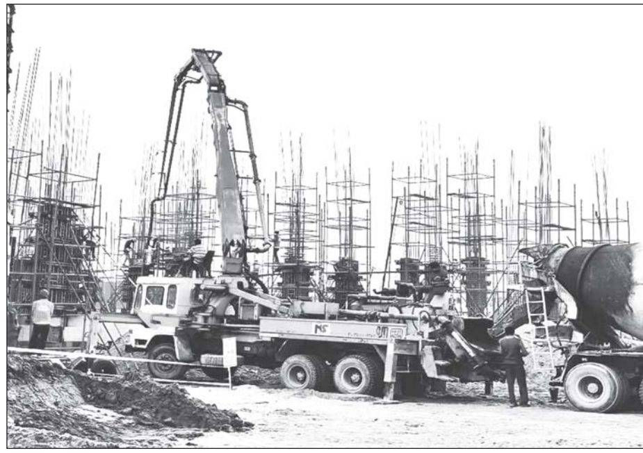
Work in full swing on site of AIIMS Jammu in Vijaypur.
