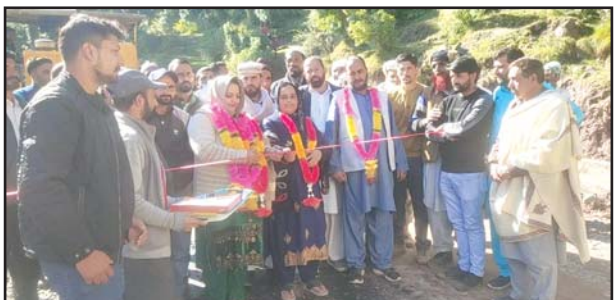
DDC Councillor Shazia Kausar inaugurating work on Koteranka-Khawas road on Sunday.
