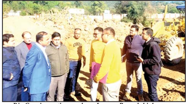
Div Com inspecting work on Jammu-Poonch highway.
