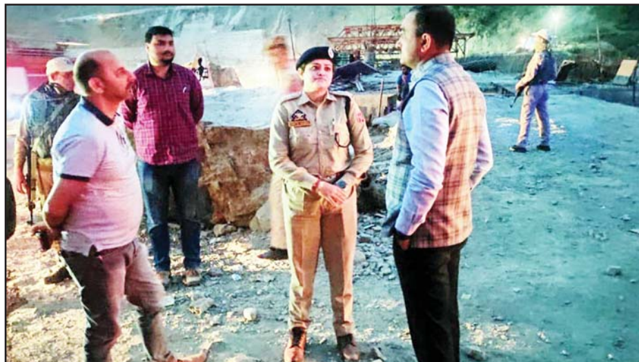
Divisional Commissioner inspecting work on NH-44.
