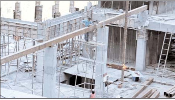
An under construction facility at Mata Vaishno Devi Ji Bhawan.
