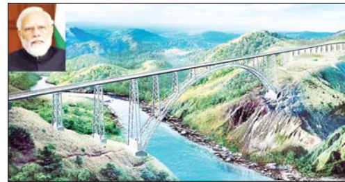
A view of under construction bridge on Chenani-Sudhmahadev National Highway.
