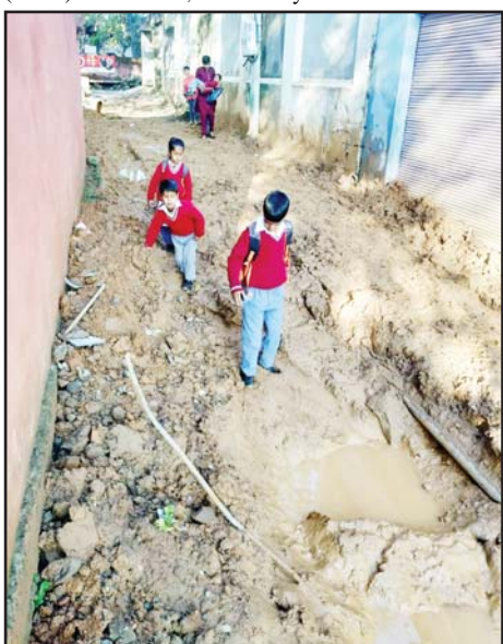
Children walking on extremely damaged Nagrota road to reach school. — Excelsior/K Kumar
