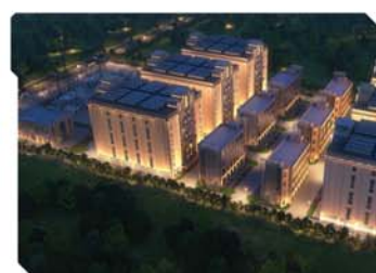
DATA CENTER HUB
