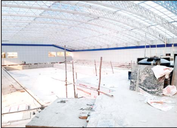
A view of under construction Swimming Pool at MA Stadium.
