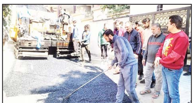
JMC Councillor Suneet Raina kickstarting blacktopping work in Karan Nagar.
