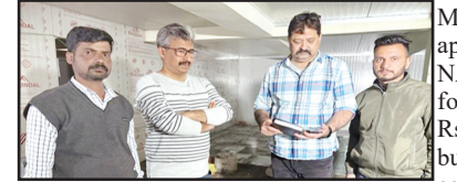
MD JK AIDCL Dr Arun Manhas during a visit to the construction site at Chenani.
