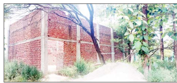
A view of incomplete Badminton Sports Stadium at Arnia.
