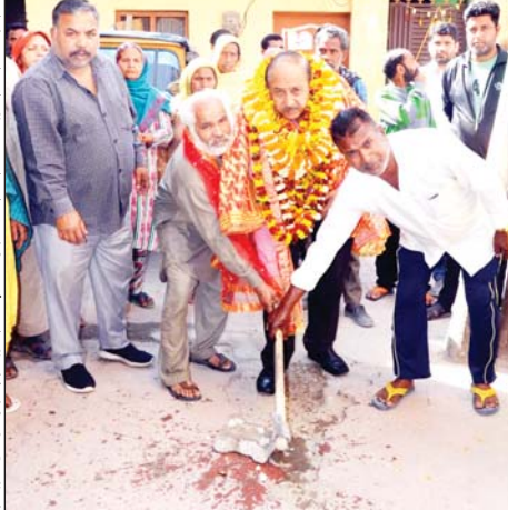
Councillor Sham Lal Basson starting lane and drain work in Ward 48 on Wednesday.
